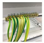
nVent ERICO Connecting, Earthing and Neutral Busbars are used to connect several earthing conductors within a panel and can be used in a variety of different applications including switchgear and control equipment, electrical equipment, for wind and solar power generation and in data centers.
